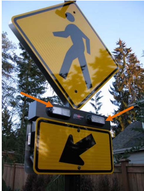
Figure 4. RRFBs are mounted under pedestrian warning signs. The orange arrows point to the RRFB lenses.
